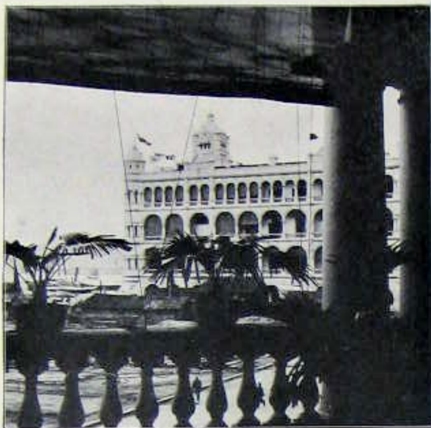
A NEW BUILDING
